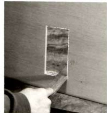
Square the Corners of the Openings
