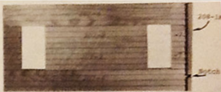
Porch Wall 2nd Floor
