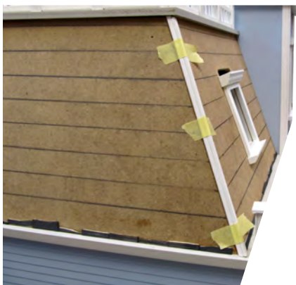
Shingle Boards and Starter Course
