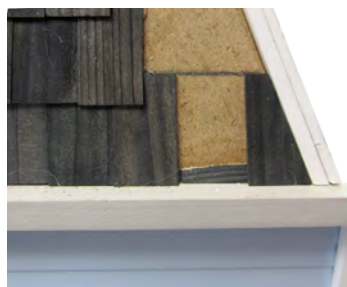
Cut the angled shingle first, then fill in
