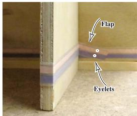
Eyelets must be installed where they can be centered on both wires.
